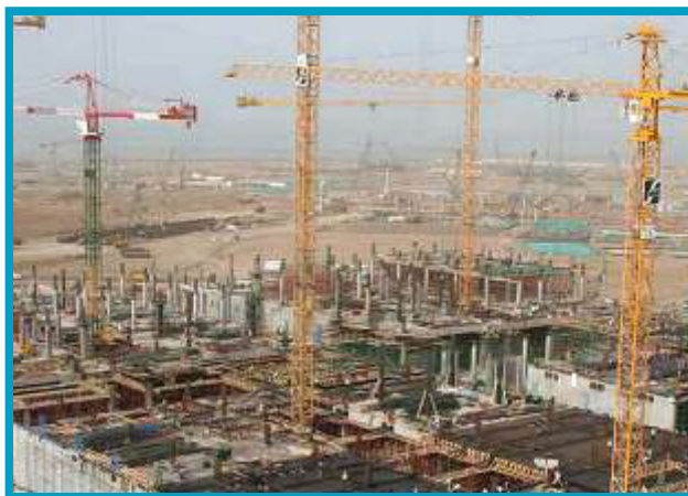
Construction progresses on the KAUST campus, March 01, 2008
